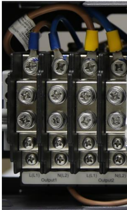
Figure 5-27 Output terminals of the AC PDU
