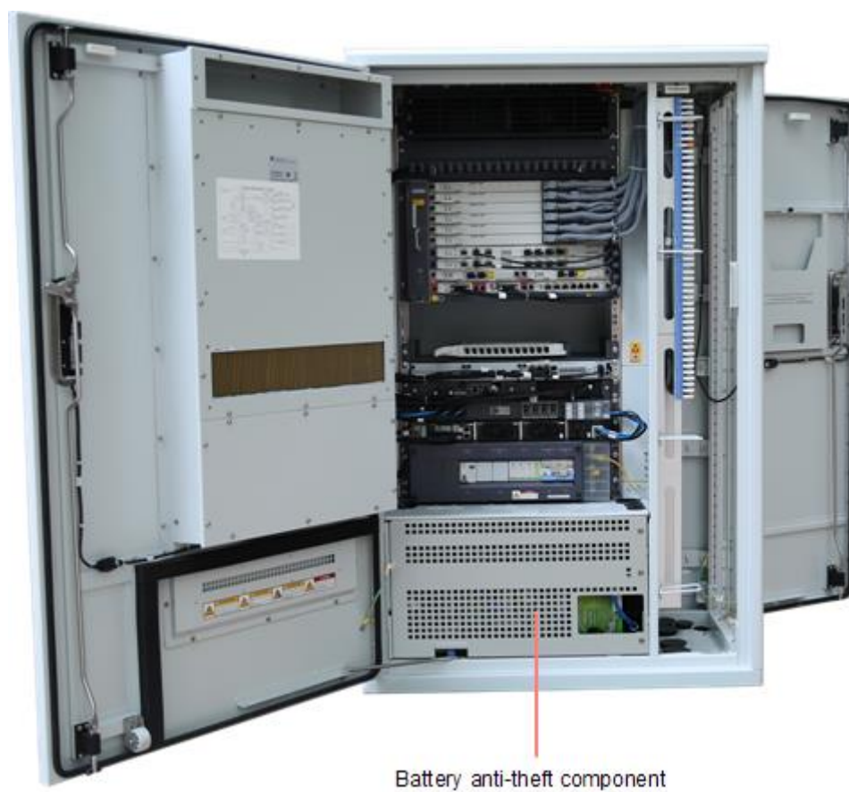
Figure 3-11 Battery anti-theft component
