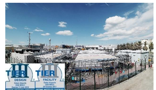
Dubai Airport, 100 racks
