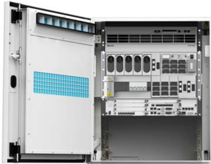
Figure 2-11 Internal structure of an APM30H (Ver.E) cabinet
