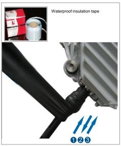
4. Using the outdoor bundling strap to bind the PVC tape tight at both ends
