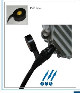
2. Wrapping three layers of waterproof insulation tape
