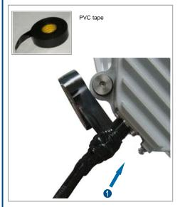
3. Wrapping three layers of PVC tape over the waterproof insulation tape
