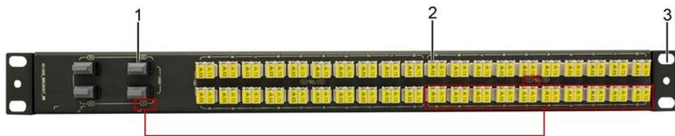
Figure 12-5 Mapping between MPO and LC adapters
